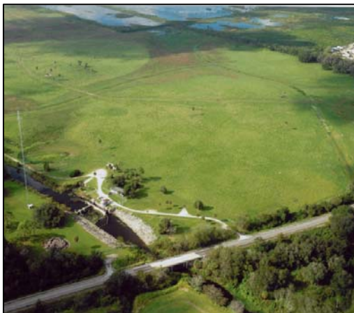
NuRF Site, October 4, 2007, pre-construction
