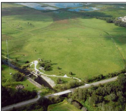
NuRF Site, October 4, 2007, pre-construction
